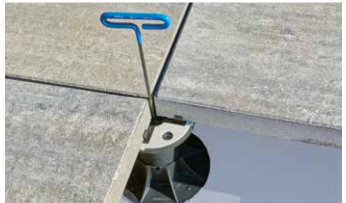
Precise leveling using adjustment key
